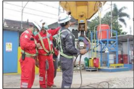
Gambar 11. Pengecekan Webbing Sling yang digunakan Sumber : Dokumentasi Proyek Bandung Advanced Science and Creative Engineering Space (BASICS) (Paket 3)
